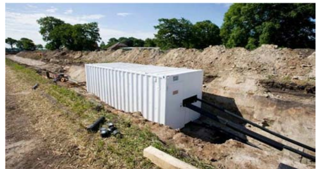
Figure 3: Specifically built container for underground cable jointing.
