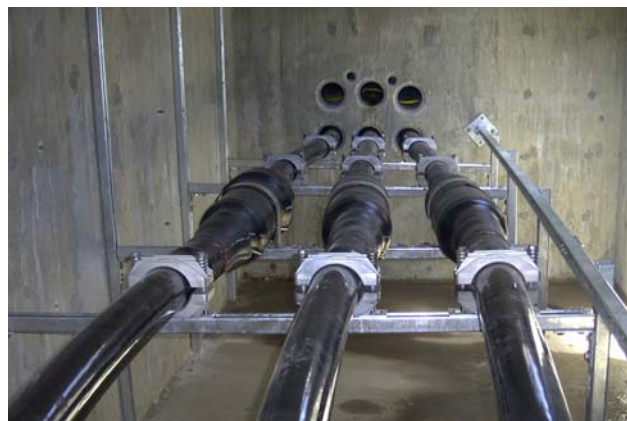
Figure 1: Rigid installation of Click-fit joints a manhole.
