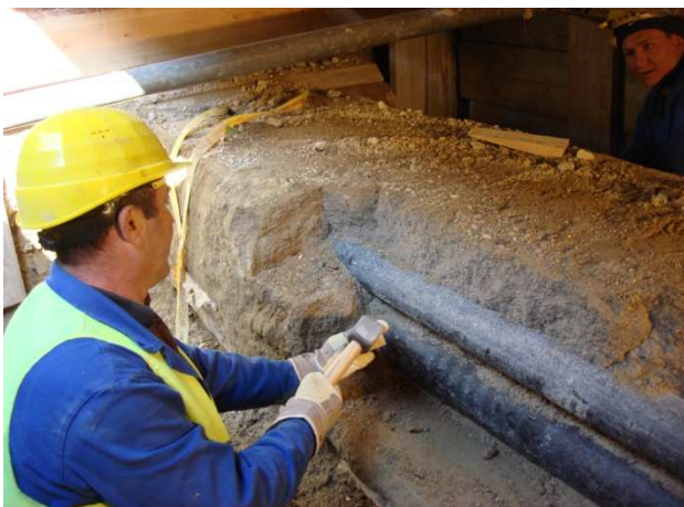
Fig.1 Removing backfill material with wooden wedges
