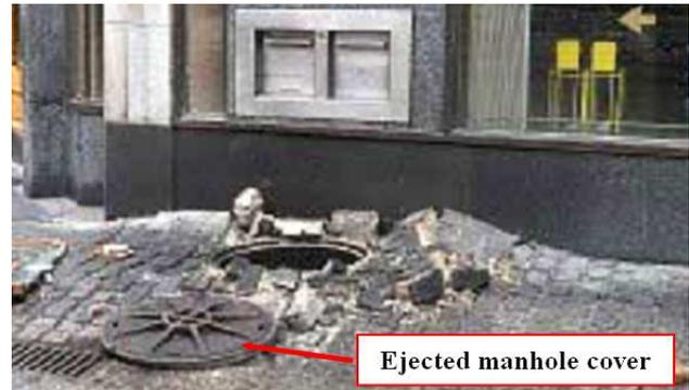
Fig. 1: Explosion in an underground vault
