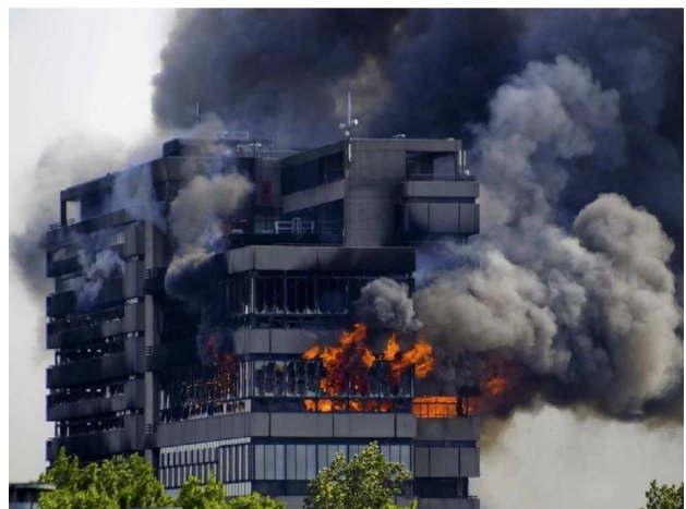
Fig 1 : Reaction to fire mainly deals with heat release, fire spread and production of smoke and gases
