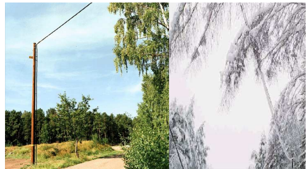
Fig.2. Universal cable from coming up from ground and with snowy branches on
