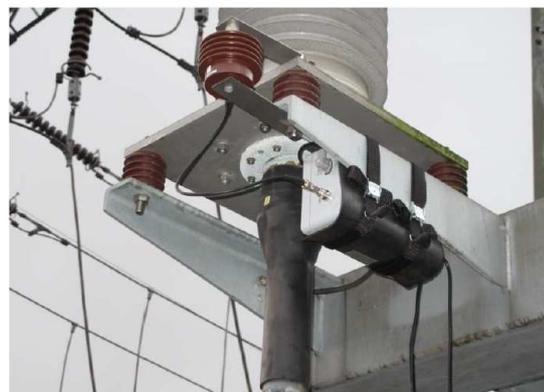
Fig. 1: Installed sensor and pre-amplifier.
