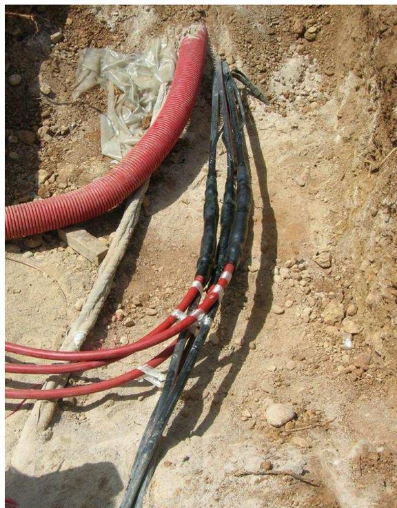
Fig. 2: 24kV Branch Joint
