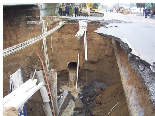
Figure 3. Photo of the cable tunnel collapse scene
