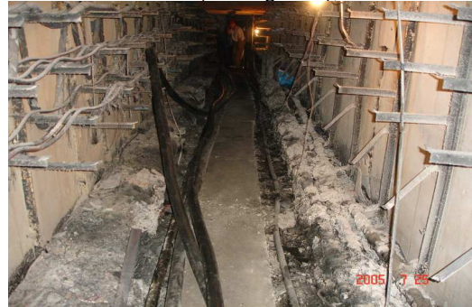
Figure 1. Photo of the power cable tunnel scene
