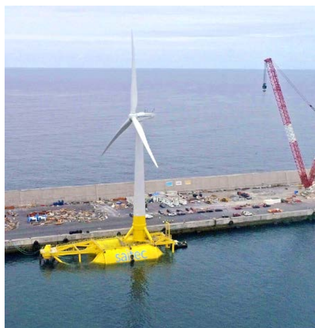
Fig. 2: 2MW full-scale floating windmill demonstrator
