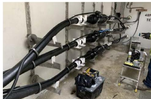
Figure 2 : Joint in manhole for single feeder
