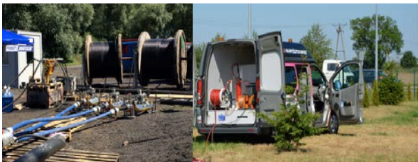
Fig. 1: Examples of (a) Watucab (WATER TUBE CABLE) technology used for the cable installations and (b) Damped AC Voltage (DAC) system applications for commissioning newly installed cable systems.
