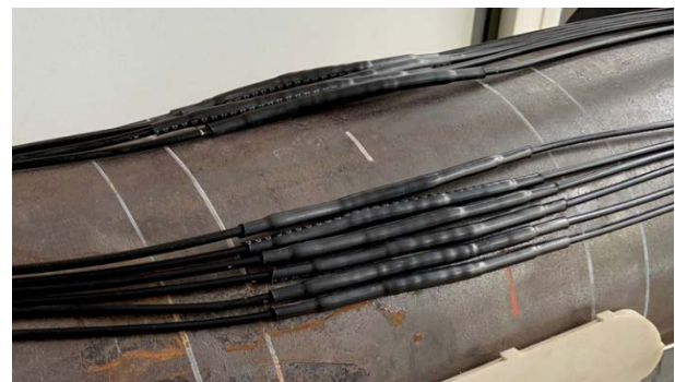
Fig. 2: Splices positioned on the inner pipe.
