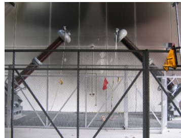
Land/sea cable interface on the French shore
