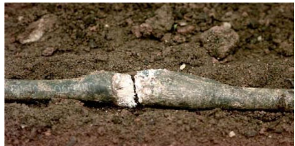
Figure 1: Corrosion Failure of Traditional 600 V Cable
