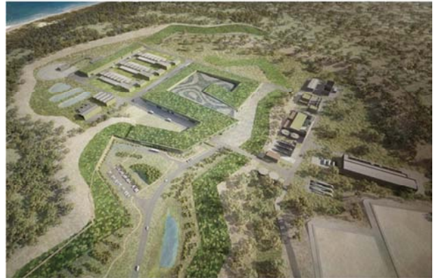
Figure 2: Victorian Desalination Plant
