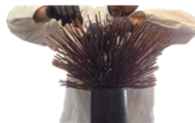
Fig. 2: Spreading out conductor wires enabling proper cleaning of wires
