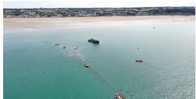
Fig. 1 Aerial view of an export cable landfall pulling
