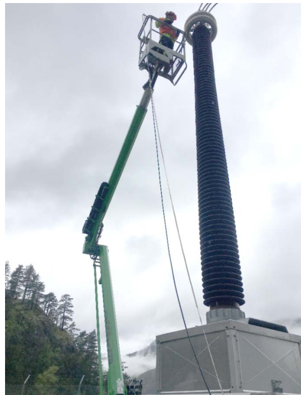
Fig.1: TDR test lead connection at dizzy height
