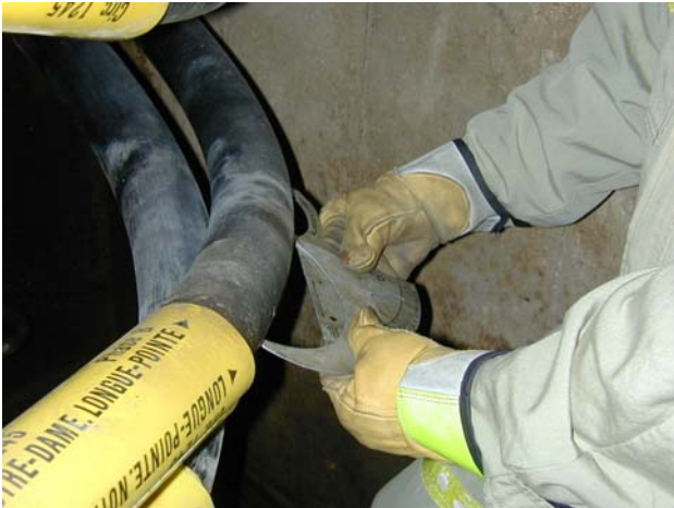
Figure 6: Measuring bending radius during inspection
