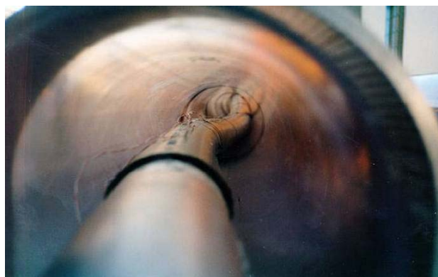
Figure 2: Snaking of a loaded HV cable inside a duct.
