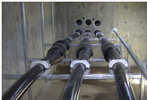
Figure 1: Rigid installation of Click-fit joints a manhole.
