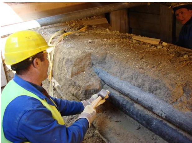
Fig.1 Removing backfill material with wooden wedges
