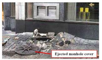
Fig. 1: Explosion in an underground vault
