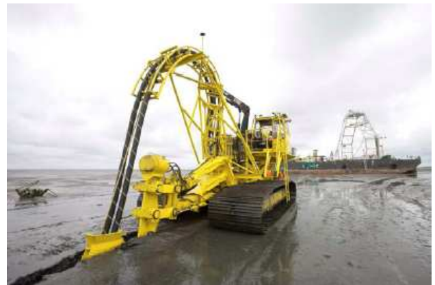
Fig. 2. Laying in progress, BorWin Germany 2009.
