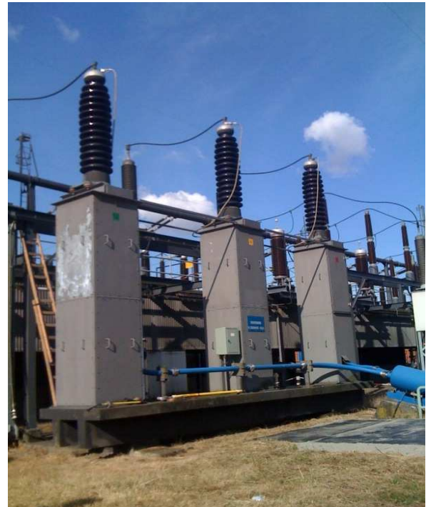
Fig 1: Service-aged HV (150 kV) gas pressurized power cable.
