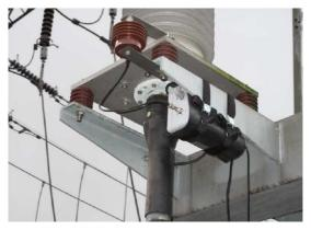
Fig. 1: Installed sensor and pre-amplifier.
