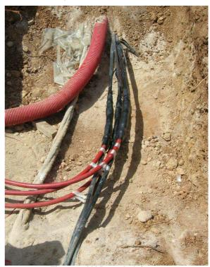
Fig. 2: 24kV Branch Joint
