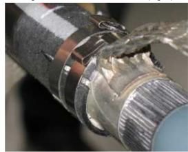
Fig. 3: Screen plate installed on the cable
