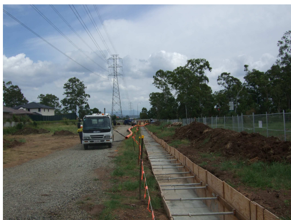
Fig. 1: The South Pine – Sandgate 275 kV Cable Corridor
