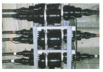
Fig.1 a 66 kV Y-branch joint
