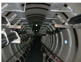
Figure 1: Site View of Shanghai 500kV Cable Tunnel
