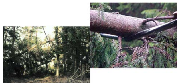
Fig.3. Fallen tree over an AXCES™ cable
