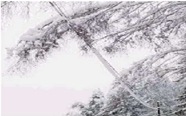
Fig.1. Heavy snow-covered branches on live cables
