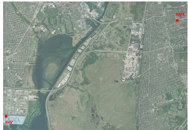
Fig. 1: Overview of the grid nodes that had to be connected with this cable project.
