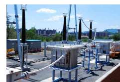
Figure 3: Four WRV systems used for 500kV 6.7km power cable tests
