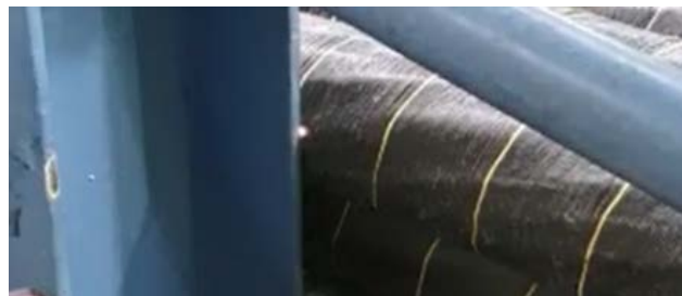
Fig. 2: Arcing during DC sheath test
