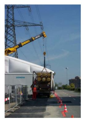
Fig. 3: Delivery of transport unit to the preassembly area
