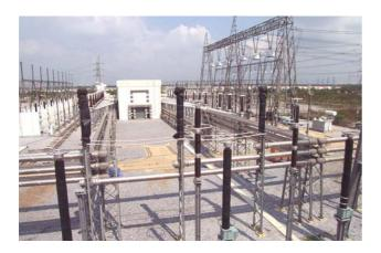
Fig. 5: Above ground installed GIL in Sai Noi, Bangkok (550 kV/4000 A)
